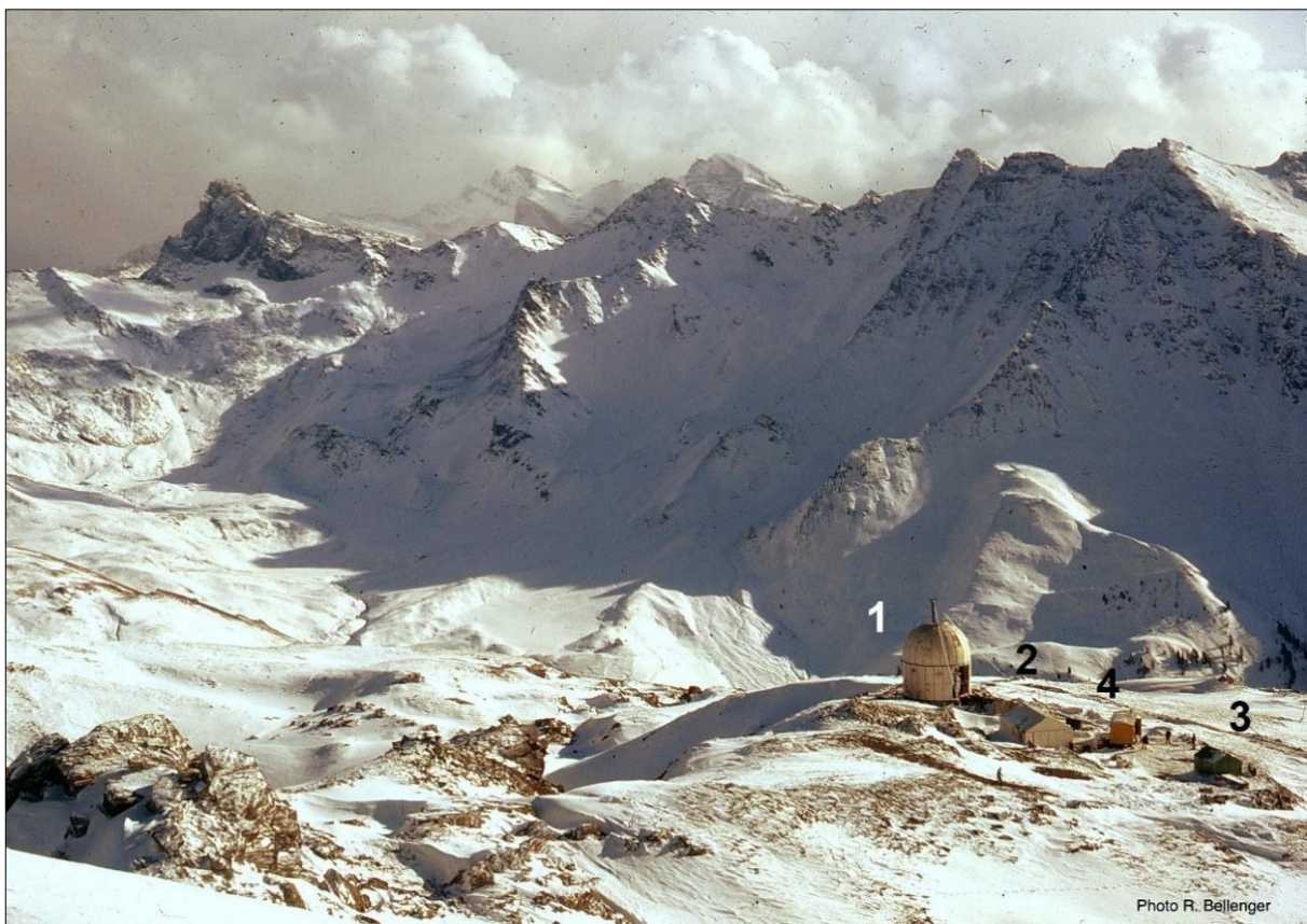
Figure 5: The observatory (2930 m) under construction in autumn 1974. One sees the unfinished 7-m dome (1), the sheet metal house (2), a hut for temporary accommodation (3) and the yellow trailer that was used by INAG for site prospection (4) (photograph: Remy Bellenger).
