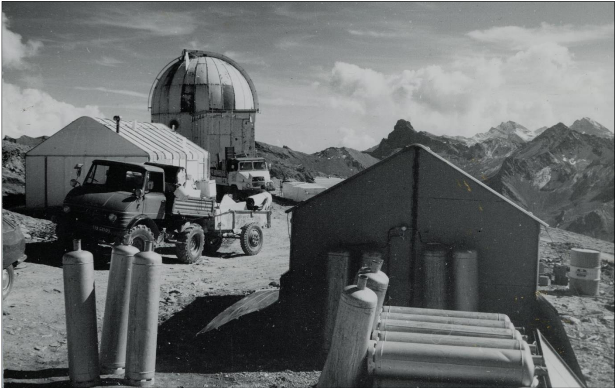
Figure 6: Building the station in the summer of 1975. The heating of the house (left) was provided by gas, and electricity by fuel generators. The Mercedes Unimog U406 at left (a 4 × 4 truck) was owned by Joseph Brunet, an inhabitant of Saint Véran who helped a lot. The shelter (at right) was temporary (courtesy: Paris Observatory).
