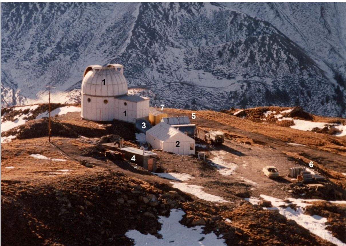
Figure 7: The completed station in 1977. One sees the two-storeyed 7-m dome and annex (1), the house (2), the double tunnel (3), the electric plant (4), the liquid nitrogen liquefier hut (5), the gas storage area (6), and the yellow trailer that was used by INAG for site testing (7) (courtesy: Paris Observatory).
